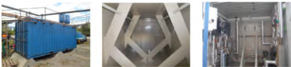
Figure 242: Standard sea-freight container as low-pressure buffer tank
