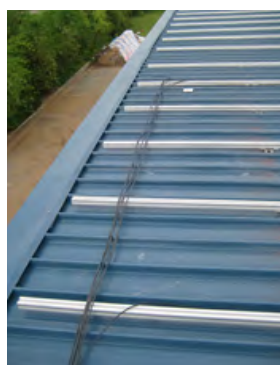
Figure 202: Prepare DC wiring within the module area and solar connector with appropriate crimping tools.
