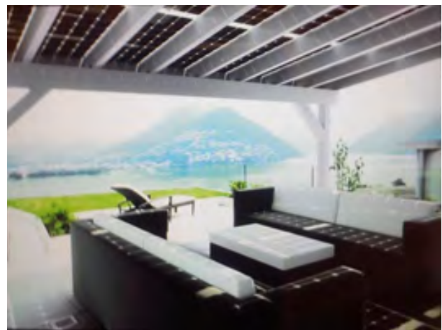
Figure 167: Sun terrace covered with semi transparent glass-glass modules for shading and power generation
