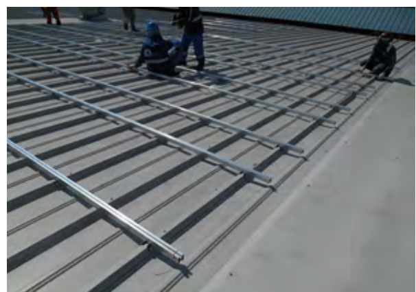
Figure 194: Support structure installation with lines to mark the edges of the profiles and tools for distance control
