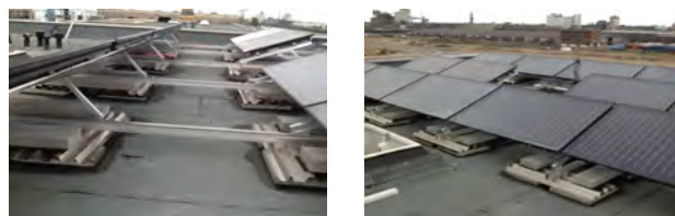
Figure 213: Roof top support structures
