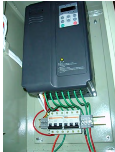
Figure 27: Solar Pump Inverter for direct connection to a motor
