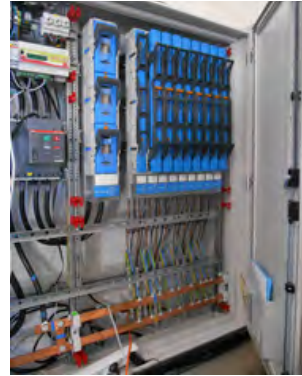
Figure 208: Installed AC connection unit
