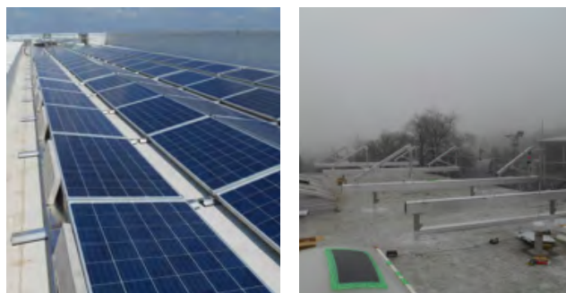
Figure 139: Flat roof installation with ballasting and fasteners
