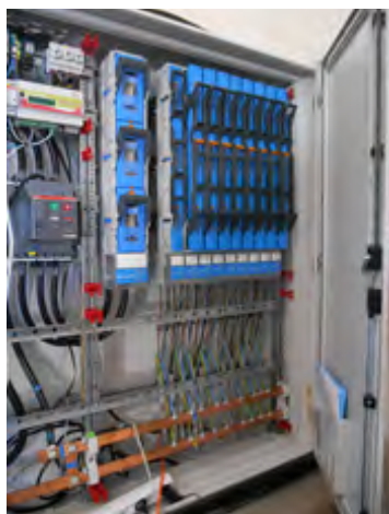
Figure 145: AC connection unit for a 250kWp solar power system with a matching transformer
