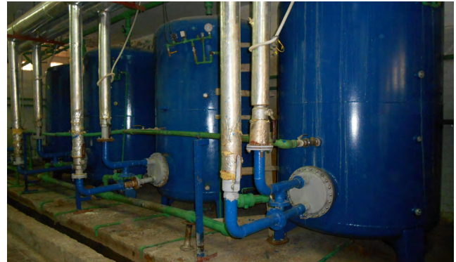
Figure 74: Complex hydraulic domestic hot water system in a touristy hotel
