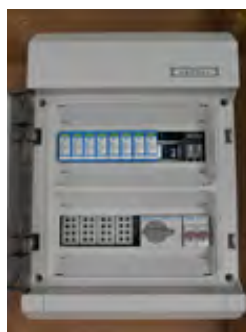
Figure 178: AC connection unit for a small size solar power system
