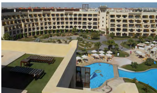
Figure 57: Large hotel unit in Hurghada, Egypt
