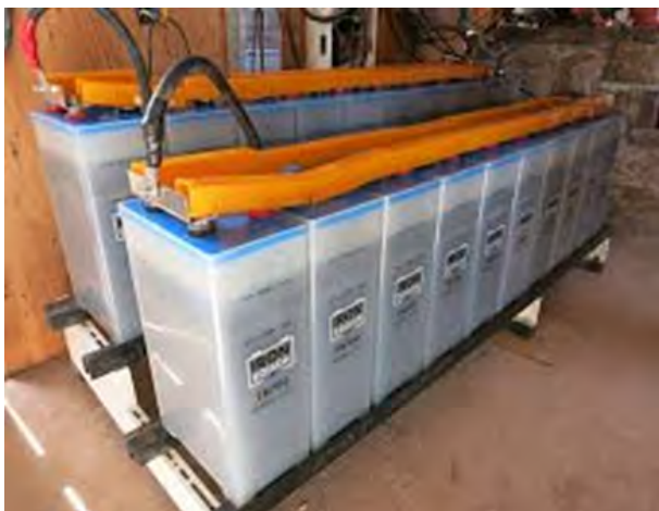
Figure 35: Nickel Iron battery
