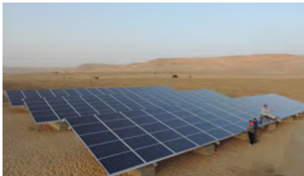
Figure 205: Installation of solar panels
