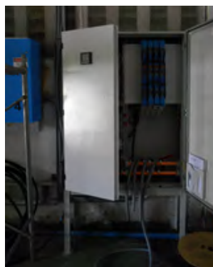
Figure 199: Installation of an AC connection unit
