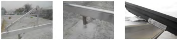
Figure 240: Support structure for a flat roof
