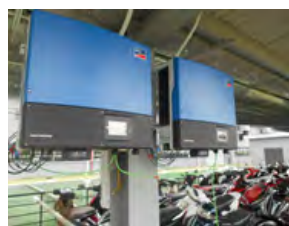
Figure 172: Different inverter installations of outside and inside solar systems
