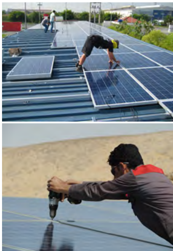
Figure 204: Assembly of PV panels
