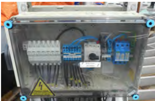
Figure 171: String combiner box in a solar power system
