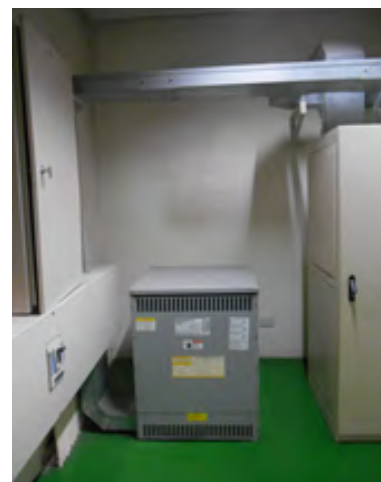
Figure 145: AC connection unit for a 250kWp solar power system with a matching transformer
