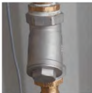
Figure 246: Dirt trap
