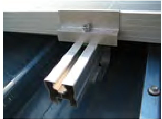
Figure 160: Standard module fasteners
