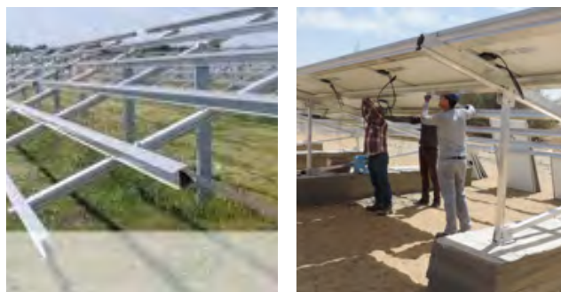
Figure 137: On-ground installations using (1) piles and (2) concrete foundations
