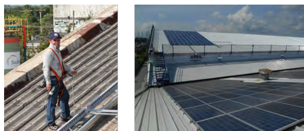
191: Personal safety equipment with a lifeline and a safety net, surrounding the installation area.
