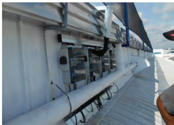
Figure 201: Installation of DC string combiner boxes
