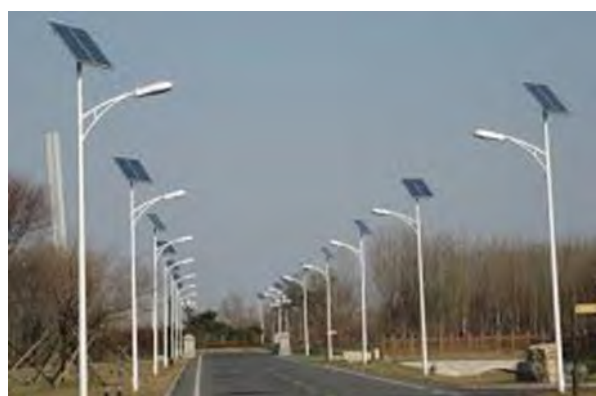
Figure 81: solar streetlight and fountain pump
