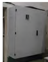
Figure 179: AC connection unit for a large-scale solar power system
