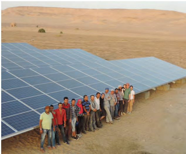
Figure 210: Finished solar power system
