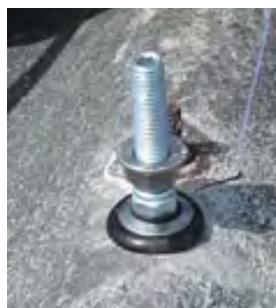
Figure 161: Support solutions for roof parallel installation
