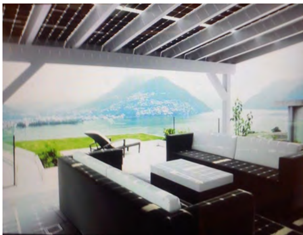
Figure 54: Shaded sun terrace with semi transparent PV modules
