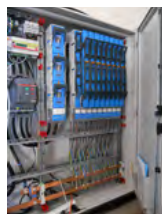
Figure 179: AC connection unit for a large-scale solar power system
